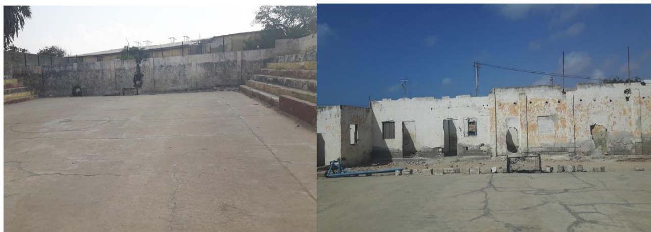
Photo 1: Theatre and Youth Sports Facility in Kismayo, selected for rehabilitation.
